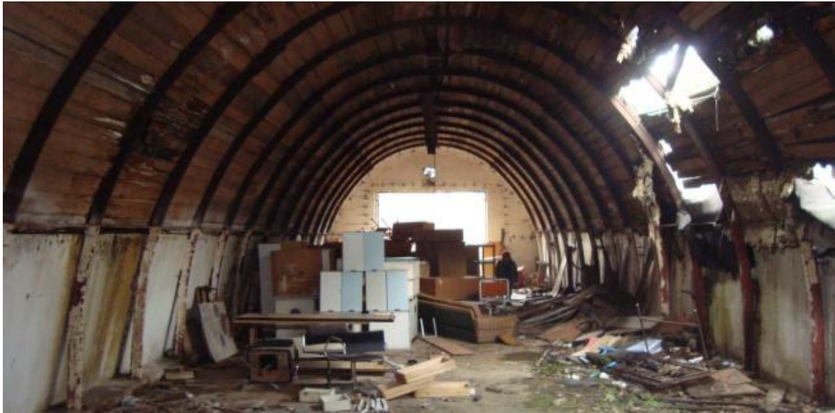
Figure 3. Building of the vegetable and fruit warehouse interior
