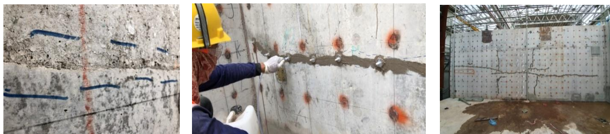
Figure 5. Repair work cold joint and cracks
