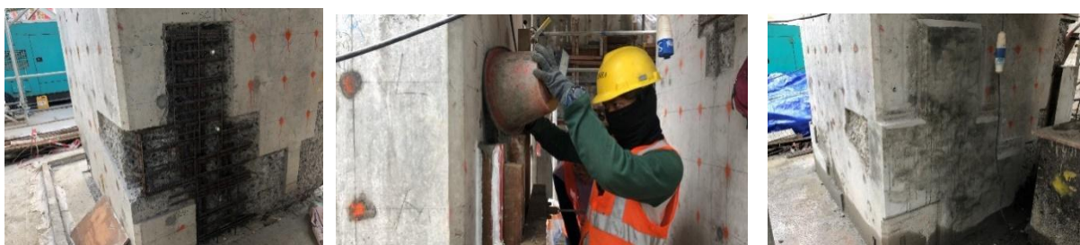
Figure 3. Honeycomb from 50 mm up to 100 mm
